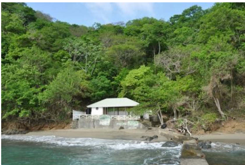
Figure 22. Rest House and jetty at Little Tobago
